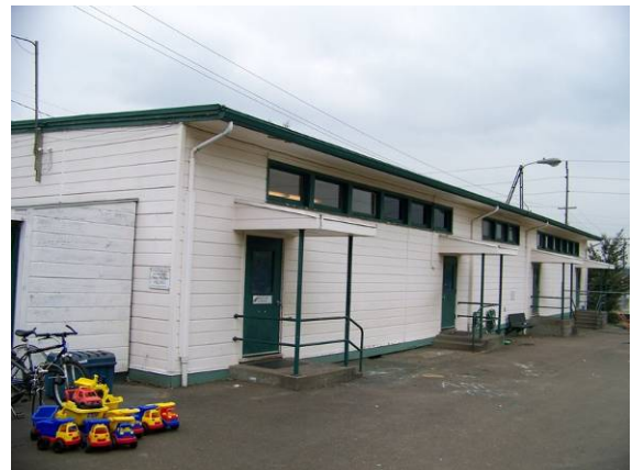
Portable (366B), west (side) and south (front) elevations, looking northeast.
