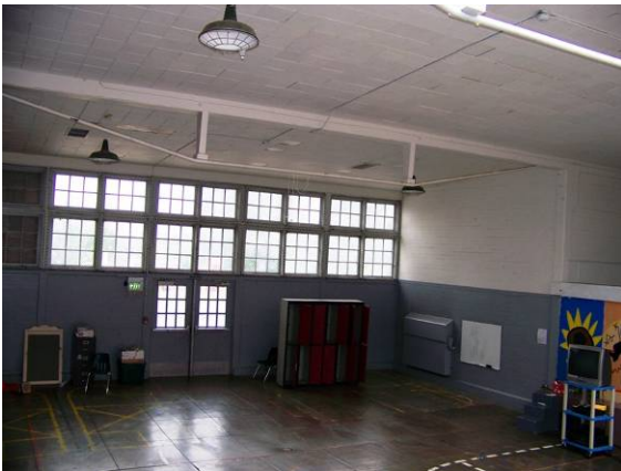
Main building (366A), gymnasium, looking southeast.
