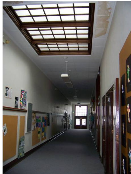
Main building (366A), south hall, looking east.
