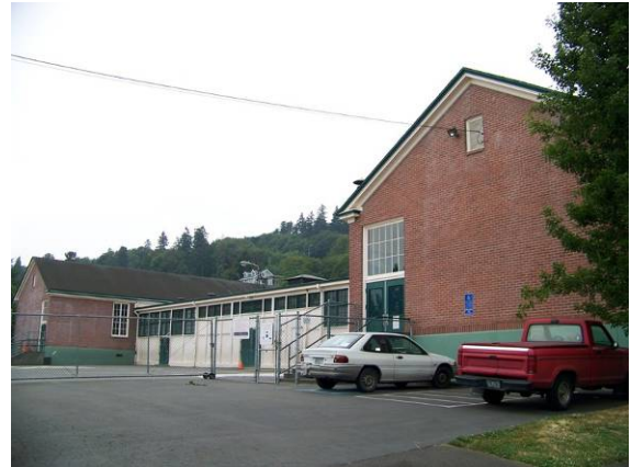
Main building (366A), east (rear) elevation, looking southwest.
