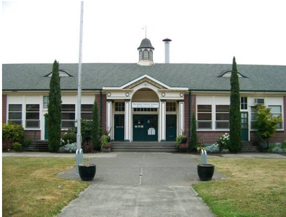
Main building (366A), west (front) elevation, looking east.
