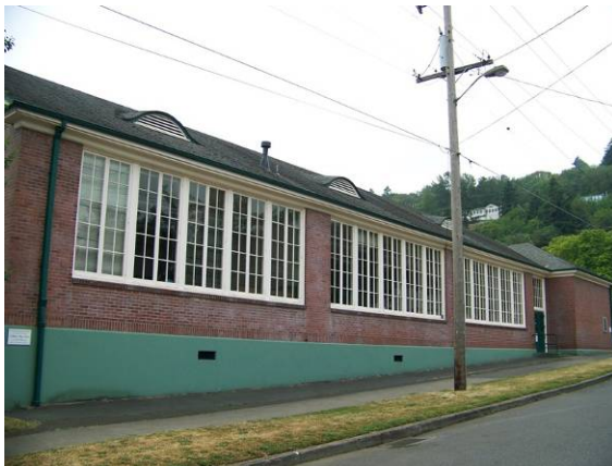
Main building (366A), north (side) elevation, looking southwest.
